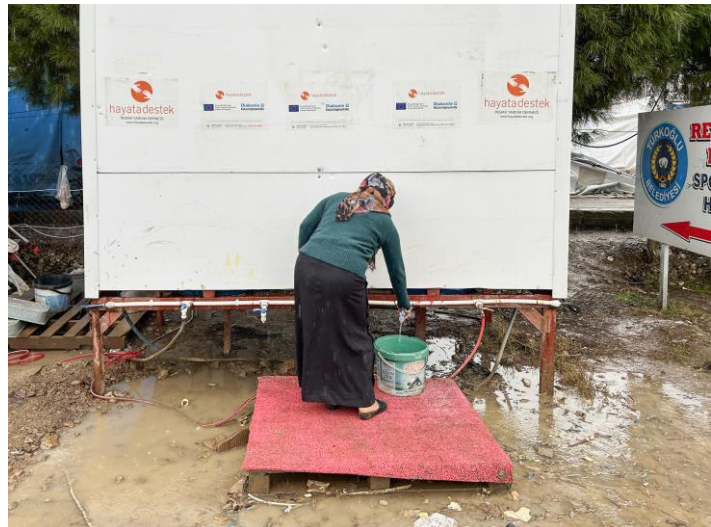
4. Water tanks installed by STL to meet the need for domestic water, Kahramanmaraş
