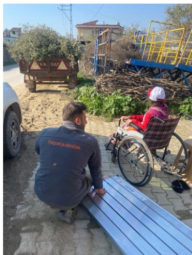
5. Disability ramp installed in shower and toilet units, Hatay
