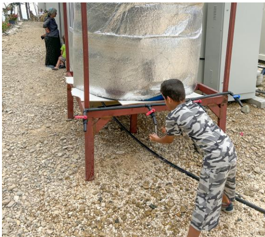
4. Water tank connected to the purifier device, Hatay
