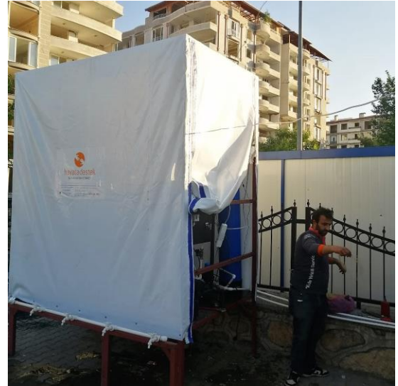
2 Water purifier installation, Adiyaman
