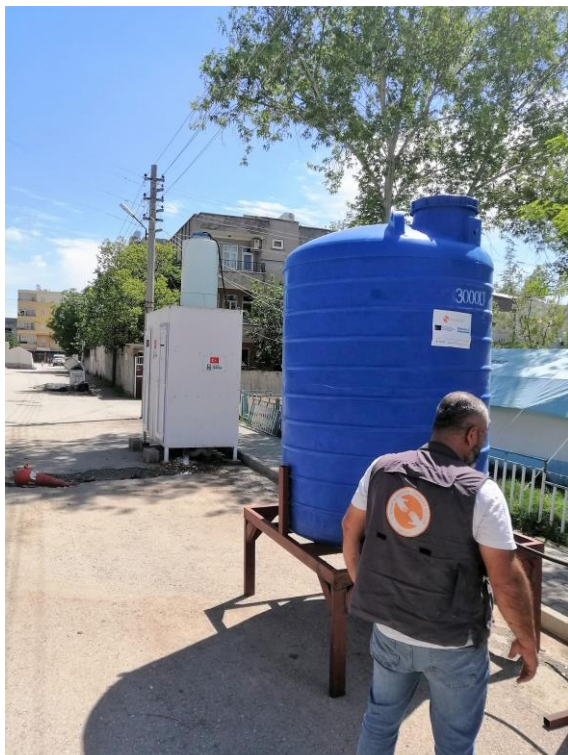
4. Water tank installation, Adiyaman
