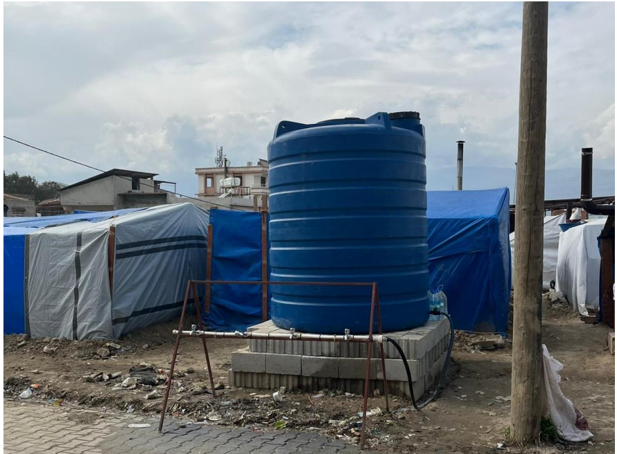
5. Water Tank, Hatay
